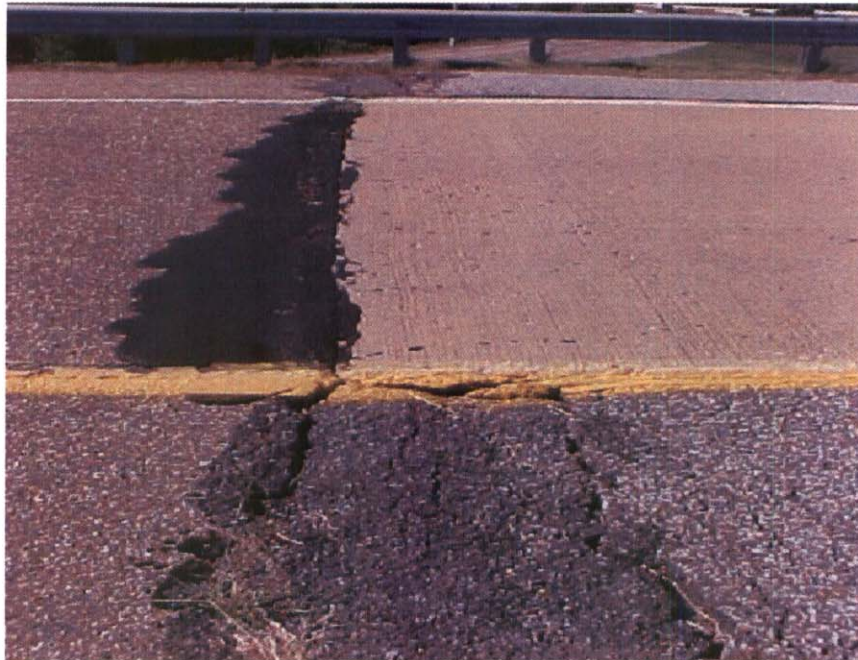
APPROACH #1 PAVEMENT SPALLING & CRACKING
